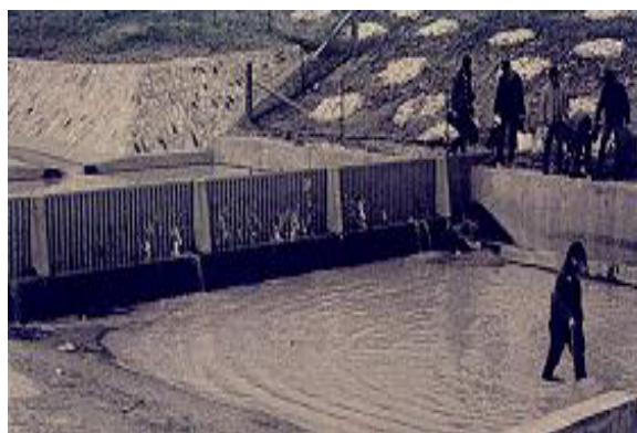
Figure 3.8 Above-ground Gross Pollutant Trap
